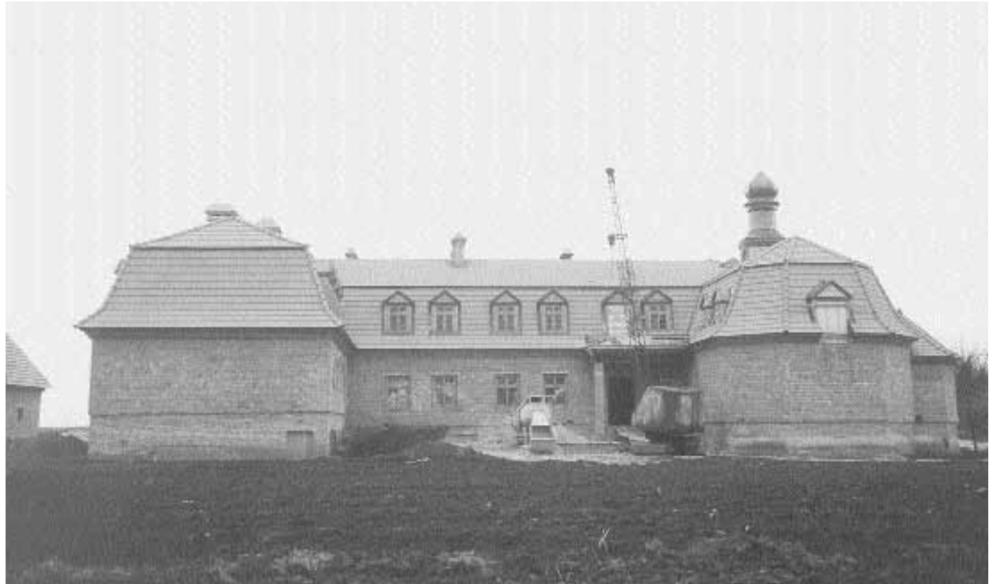
The nearly completed museum-memorial complex located in Patriarch Josyf Slipyj’s childhood hometown of Zazdryst.
