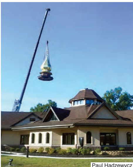
A crane lifts the main cupola for placement atop the church on Friday, September 20.
